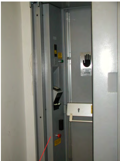
EMERGENCY PUSH BUTTON TO UNLOCK BOTH DOORS
